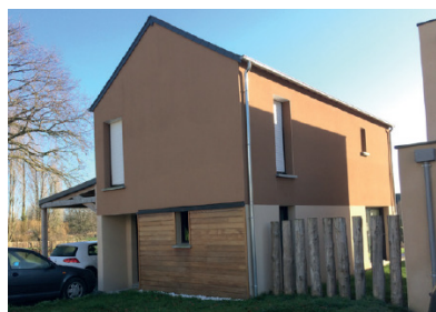
Architecture contemporaine, Servon-sur-Vilaine
